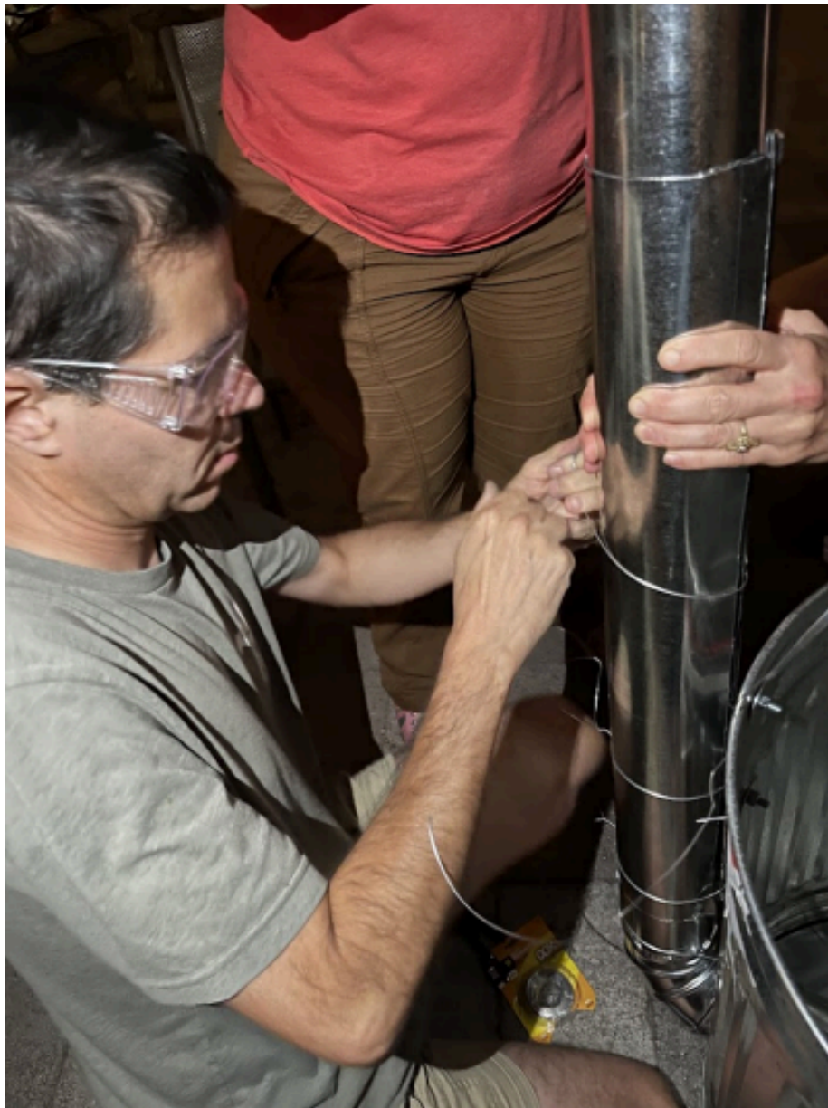
Figure 4. Chimney attachment using high-temperature wire.
